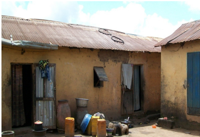
Figure 5. Cement plaster habitat in Natitingou. Source : Aikpon (2010).
